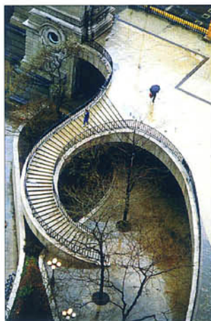
Staircase at North Michigan and the Chicago River (1983)
